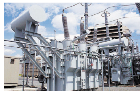
230kV Transformer
